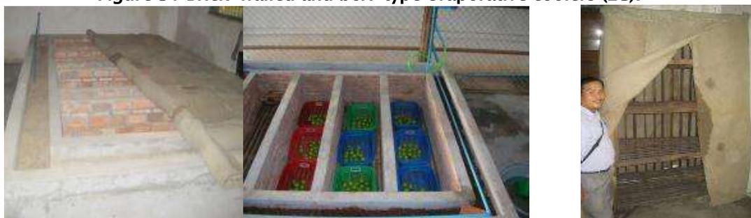
*Brick-walled EC 4.5x2.5x0.6 m in length, width & height, 15–20 cm double wall with moist sand insulation*
