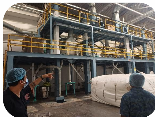
Fig 25: Inspection of SHPL hub by N+3F
